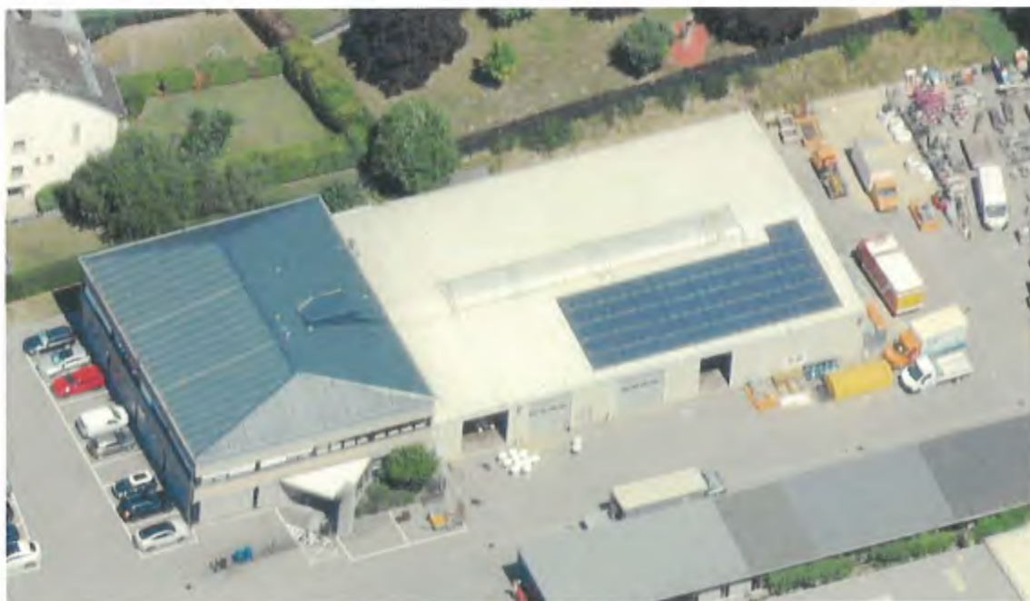
Figure 25 : Enveloppe thermique - Hall service technique
